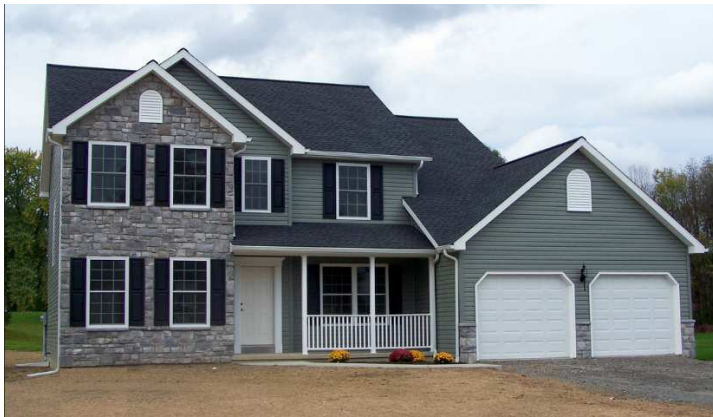
TWO STORY: Suitable on flat site where space is limited. Courtesy of finelinehomes.com
